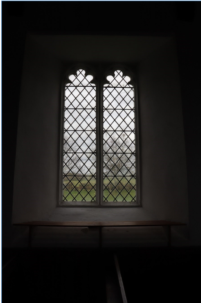
Figure 4. The view looking north across the proposed development area from within the nave of Friston parish church.
